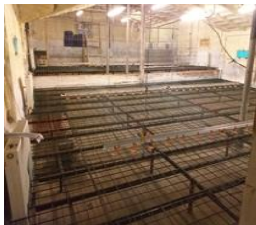
Figure 1. Installation of the stages
